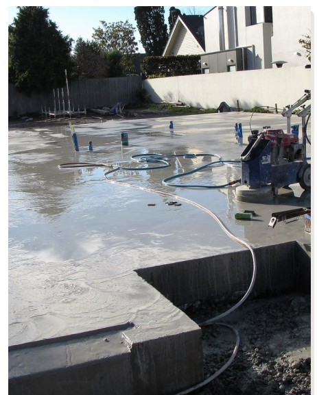
Rain-damaged slab restoration
