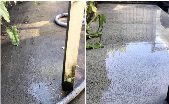
Mid depth Grind & Seal outside concrete - Before and After
