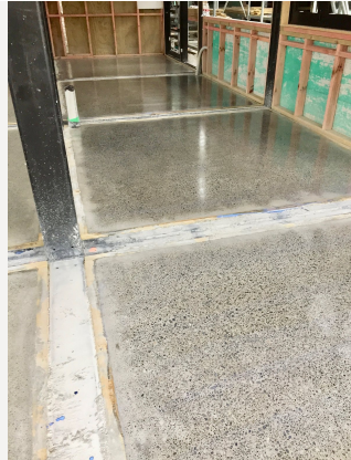
Boxed Quarter - Full depth grind with wax sealer
