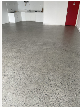
AFTER - Grind & Seal to Vape Shop
