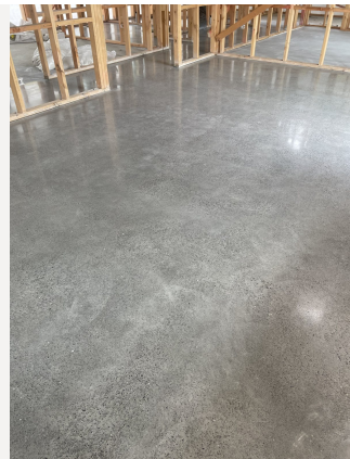
Grind and Seal Concrete Floor (Woolston)
