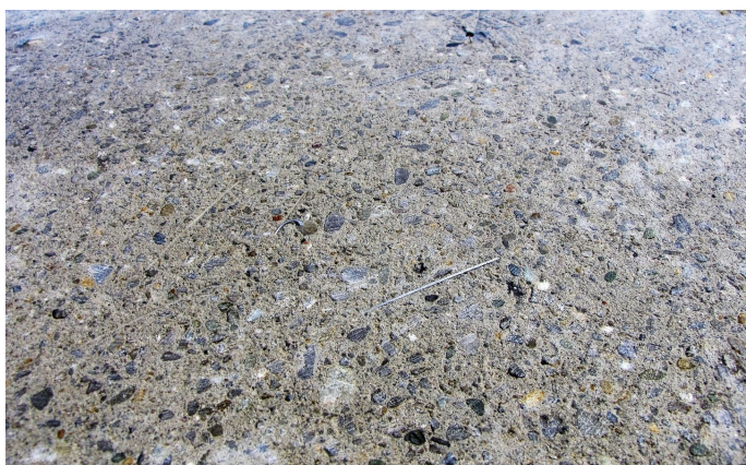
STEEL SLITHERS IN CONCRETE - EXTRA CHARGE
