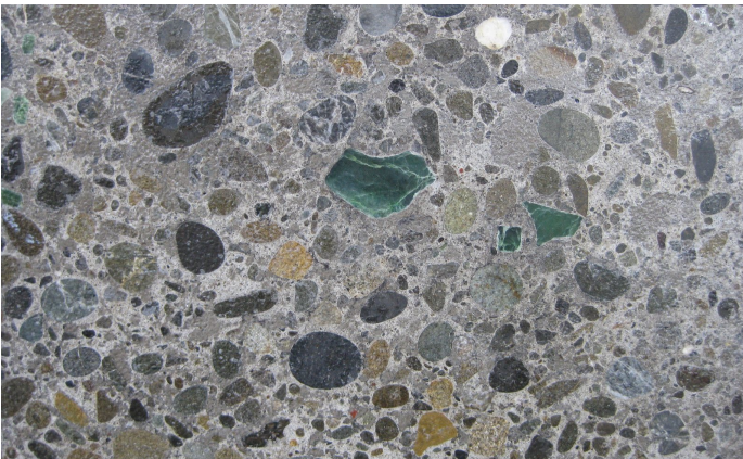
Grind and Seal Bench top with Greenstone
