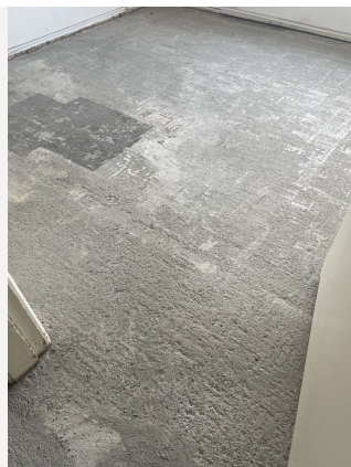
Before - Grind & Seal Concrete Floor (New Brighton Mall)
