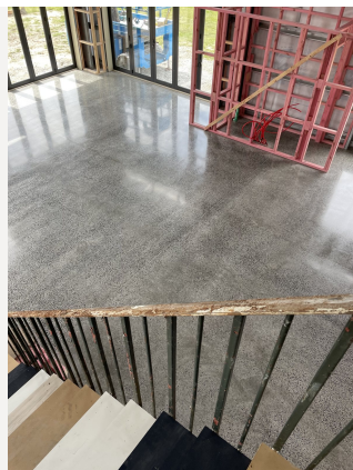
Mid depth grind to concrete with High-spec polish applied
