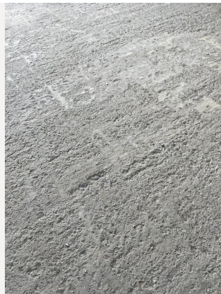
BEFORE Picture to a mid-depth Grind & Seal to very rough, old concrete floor in New Brighton
