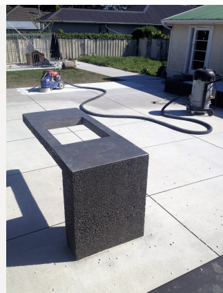
Grind and Seal Courtyard 2
