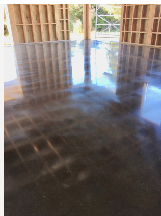
Polished Concrete Kaikoura
