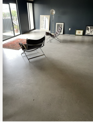
Grind & Seal Concrete Floor (Ferrymead)
