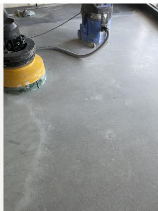
Mid-process pic Grind & Seal concrete floor
